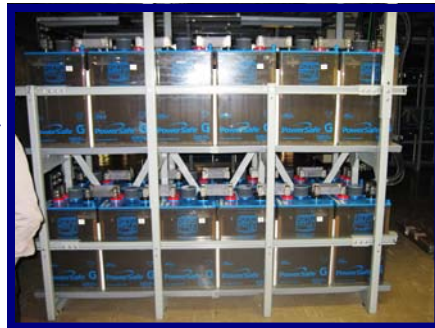
These bins hold battery acid to support “Cincinnati Bell” when the power goes out.
